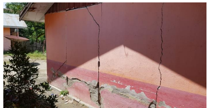
SDN Poboja Damage Reviews
