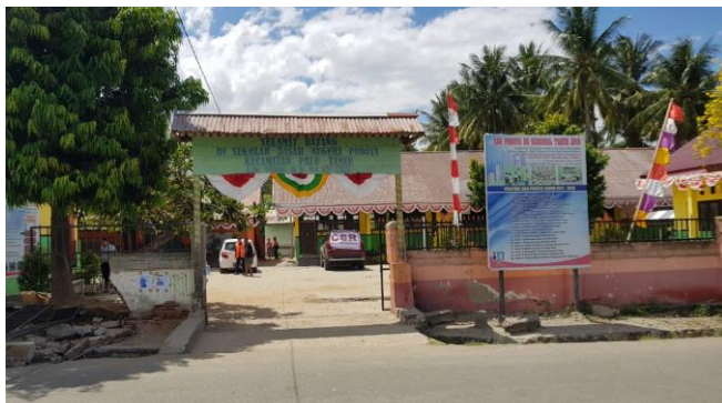
SDN Poboja Damage Reviews
