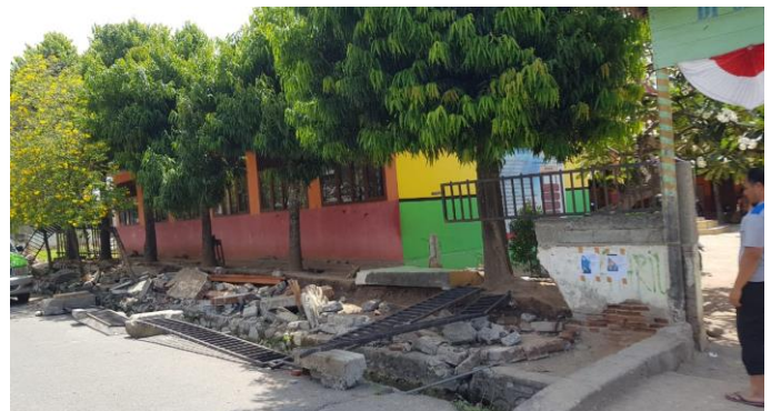
SDN Poboja Damage Reviews
